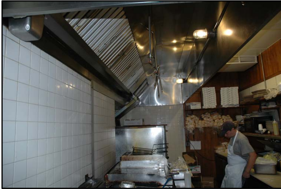
Front kitchen area with view of exhaust system (Stainless Steel Hood).
