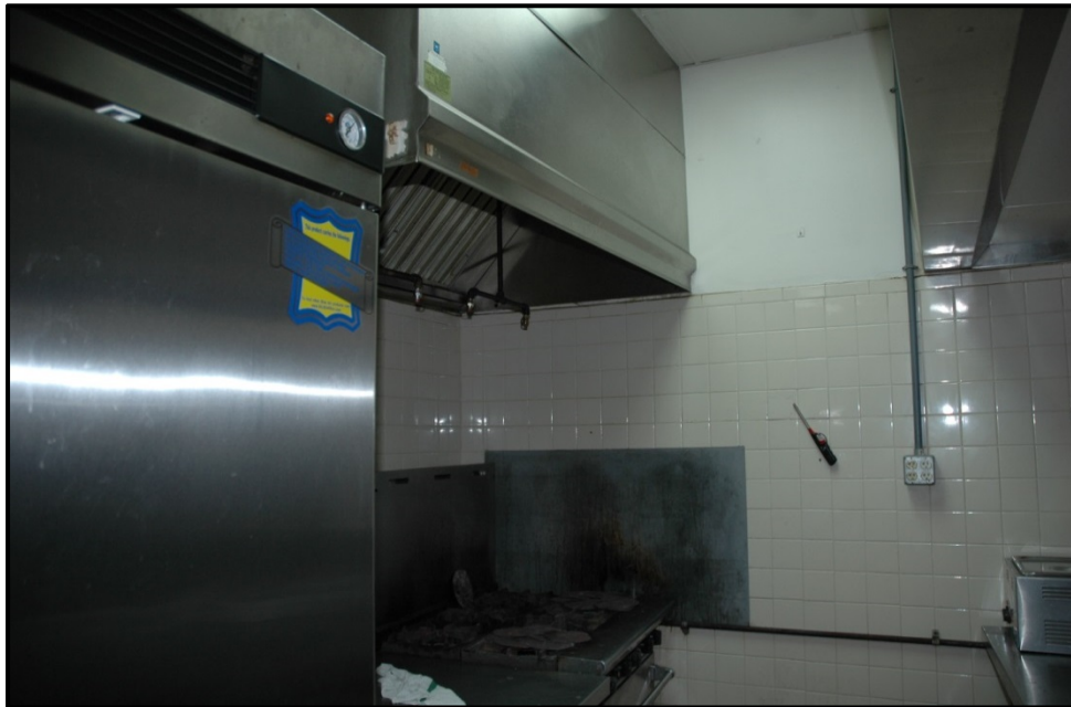
Rear kitchen area with view of exhaust system (Stainless Steel Hood).
