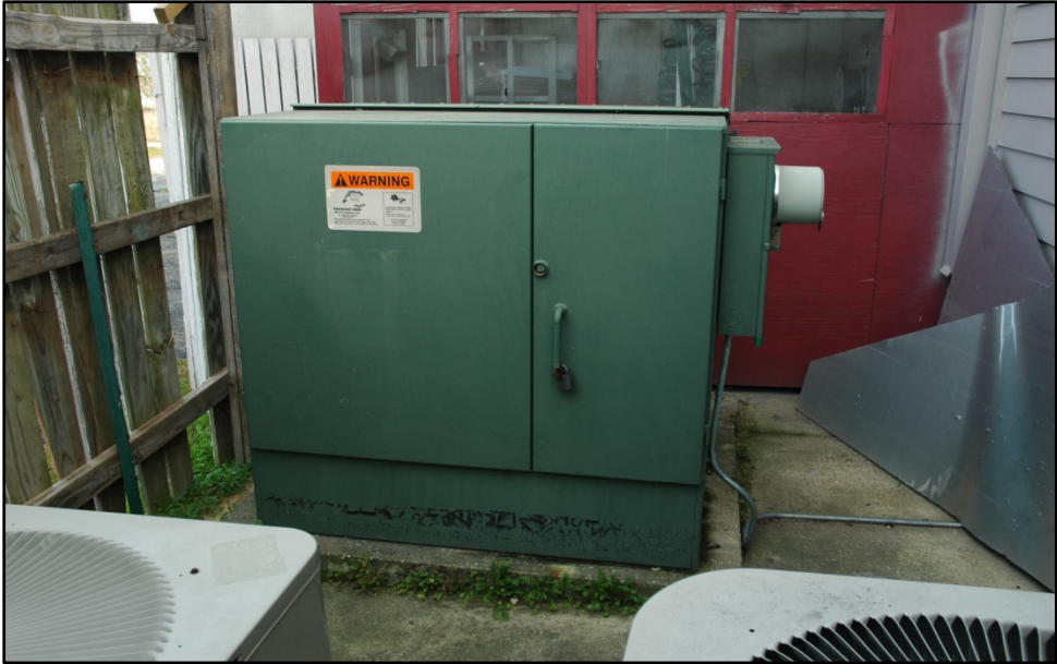
Electrical transformer owned by the City of Lumberton.
