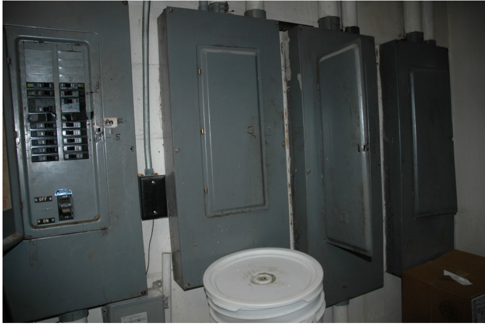
Electrical panels in storage room.
