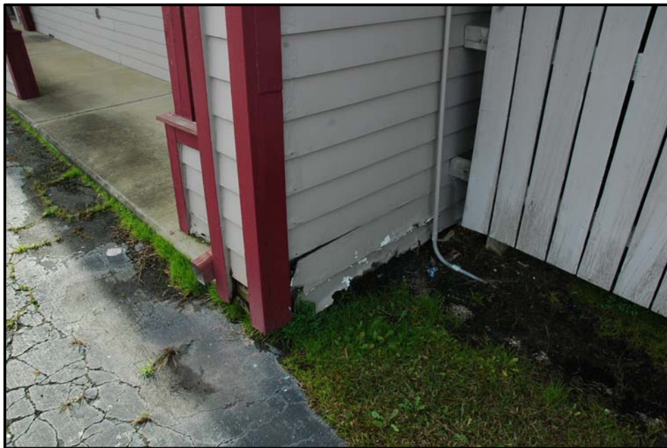
Damaged siding at northeast corner.
