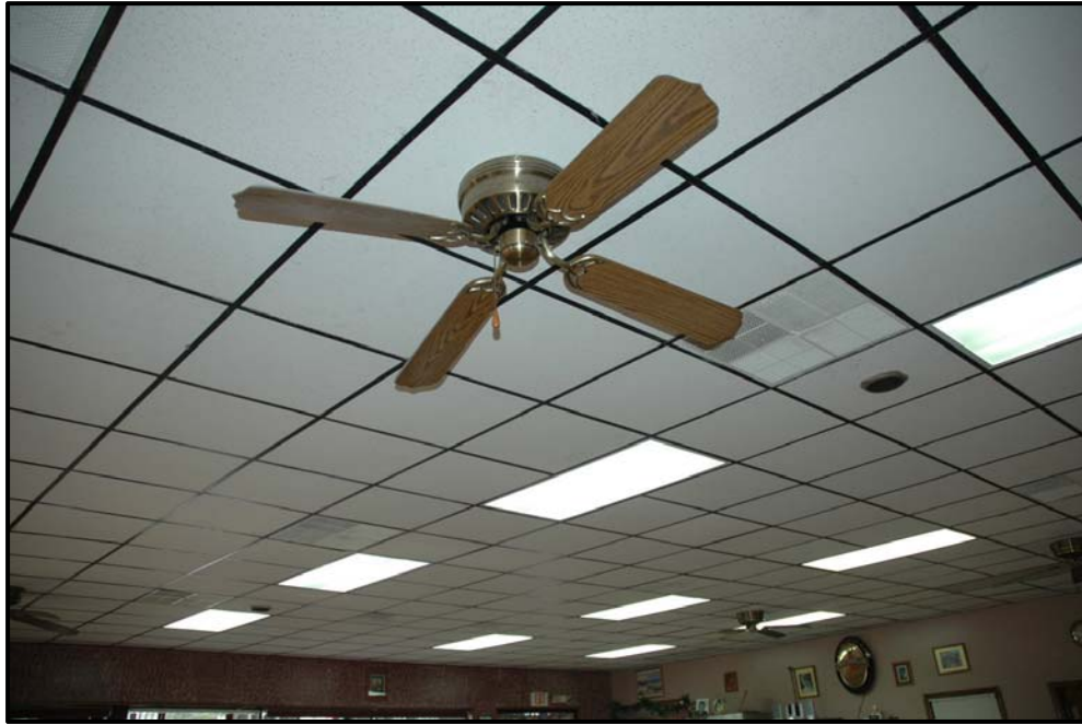
Cel-o-tex ceiling tiles with recessed fluorescent lights
