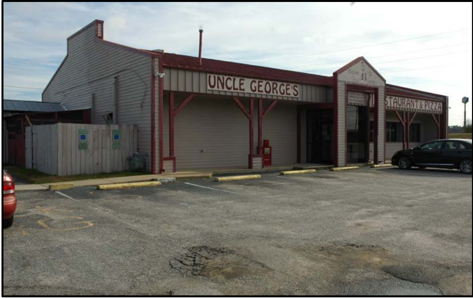
Northwest side view and front view.
