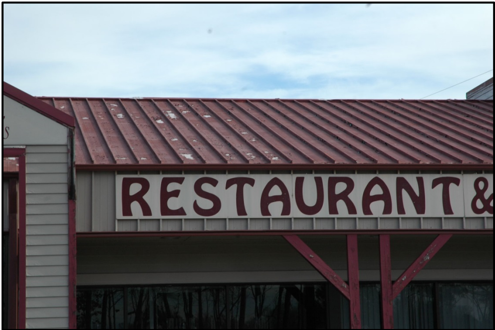
View of metal roofing.
