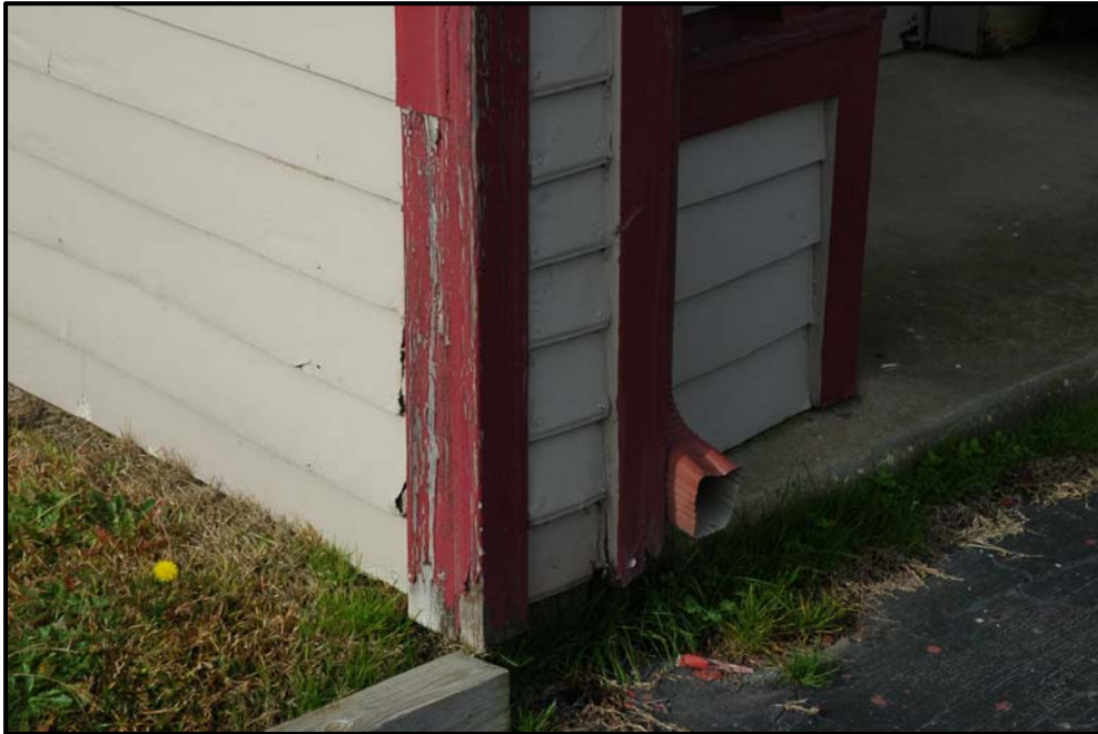
Damaged vertical trim boards
