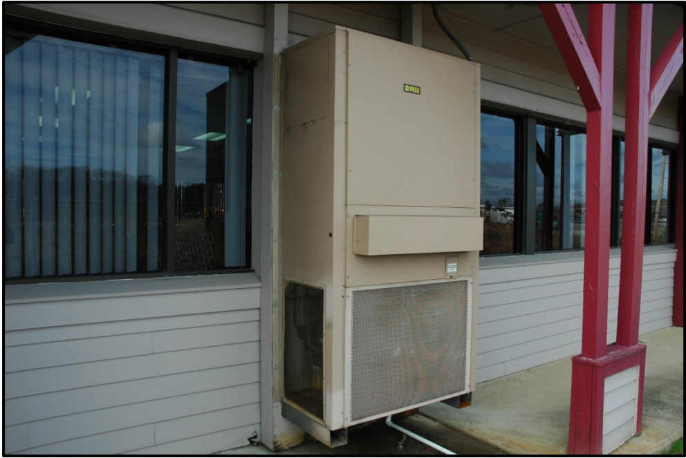
Through the wall HVAC unit
