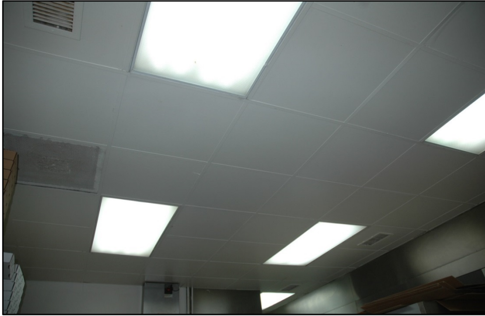
Kitchen ceiling panels with recessed fluorescent lights.
