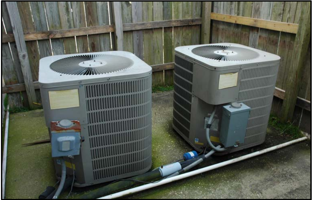
Heat Pump Units
