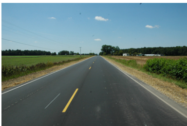
View along US 301 looking south.
