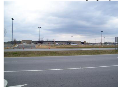
New Walmart under construction
